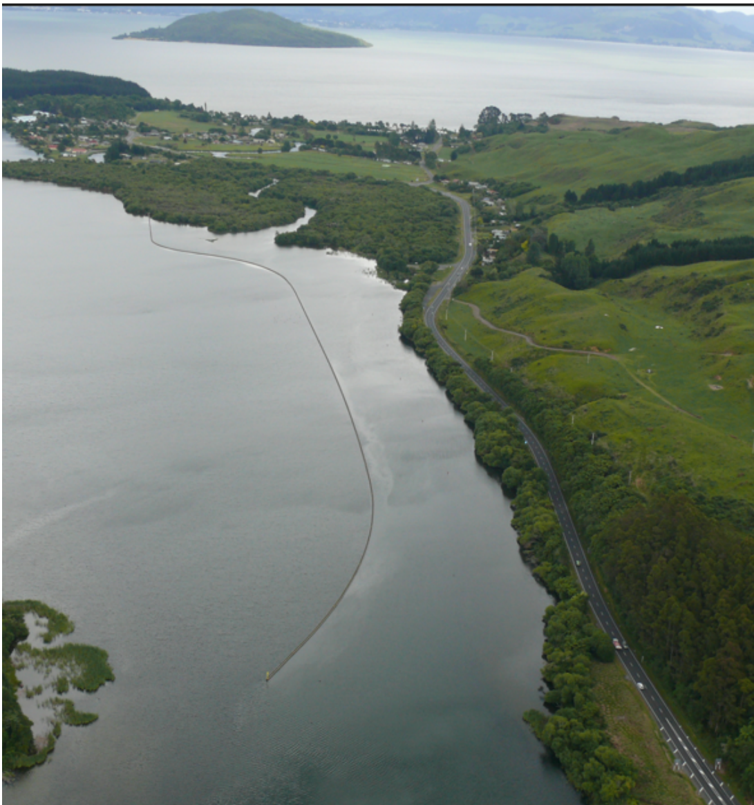
Figure 10: Aerial image of Ohau diversion wall
